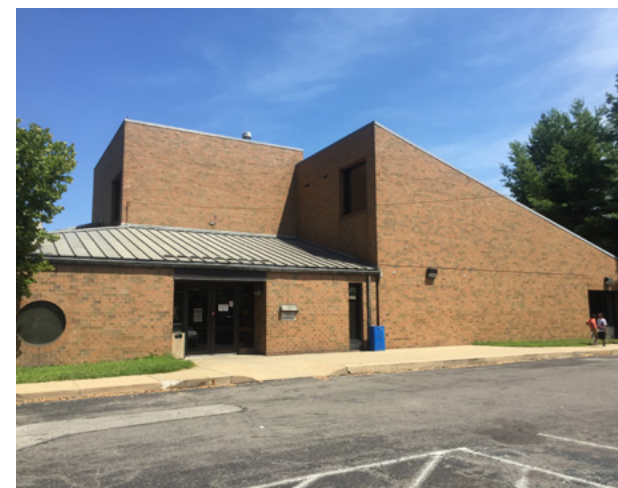
Entryway from parking lot
