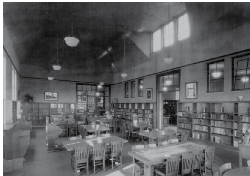
Interior Prior to Renovation- 1928
