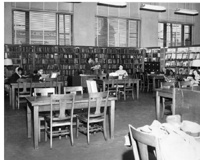
Mt Pleasant Facility Interior - 1952
