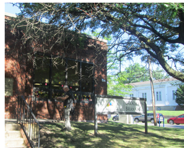
Main entry from Pearl Road
