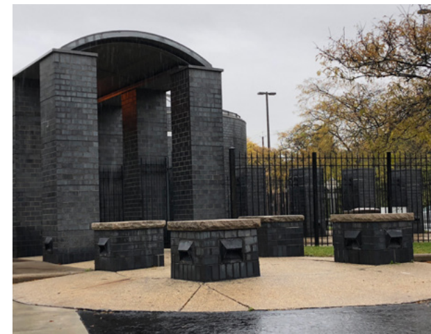
Main entrance off parking lot
