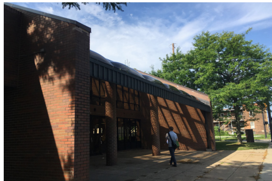
Main Entry from St. Clair Avenue
