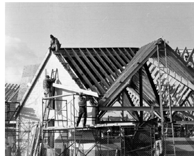
Hough under construction - 1983
