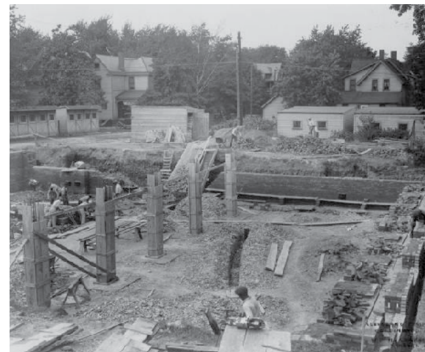
Branch under construction - 1927
