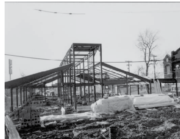
Union under construction - 1982
