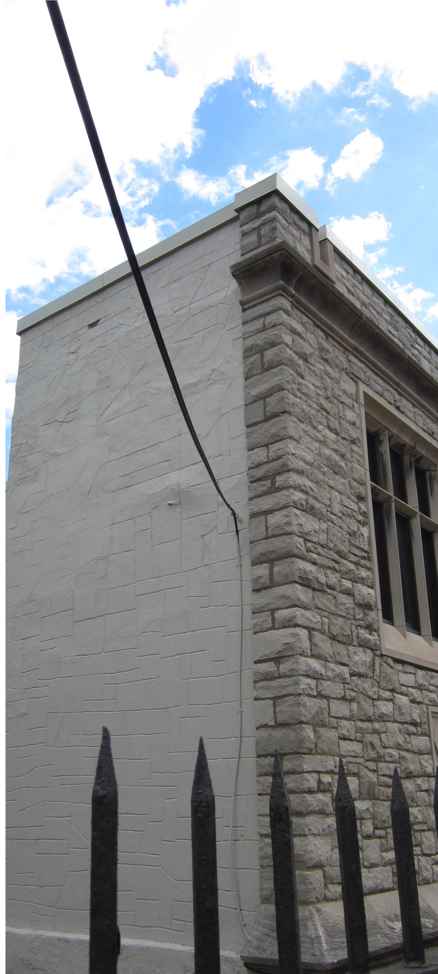
EXISTING SOUTHWEST CORNER
