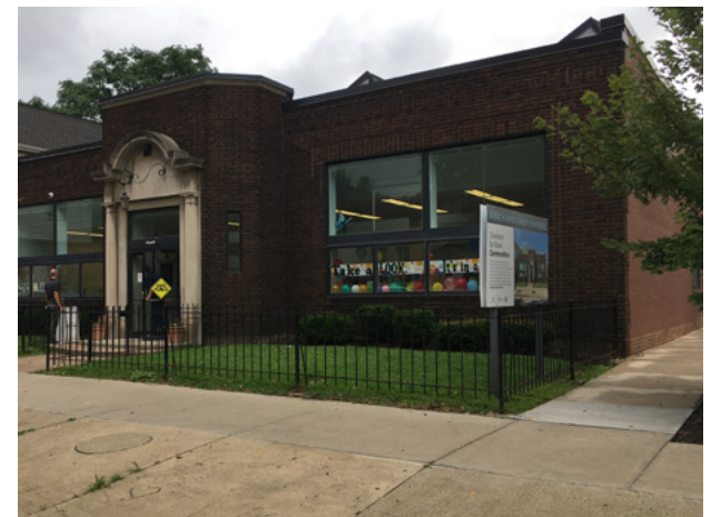
Main Entry from Jefferson Avenue
