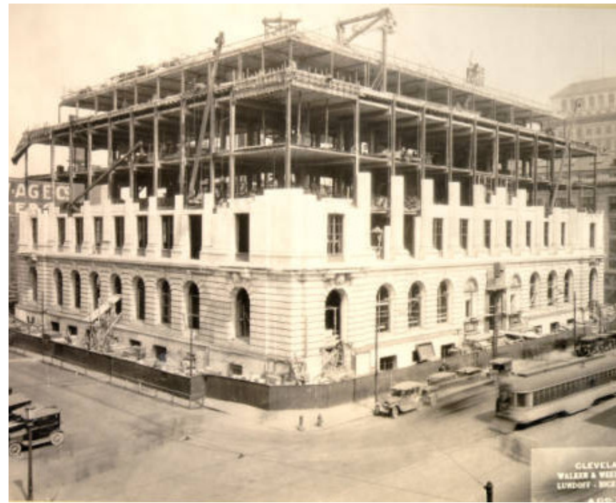
Main Building Under Construction
