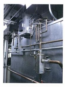
The additions of CO2 demand ventilation control (see option below) should allow the existing DriSteem humidification units to perform to the RH levels needed with reduced OA. No relocation of the DriSteem units is recommended unless set points cannot be reached.
